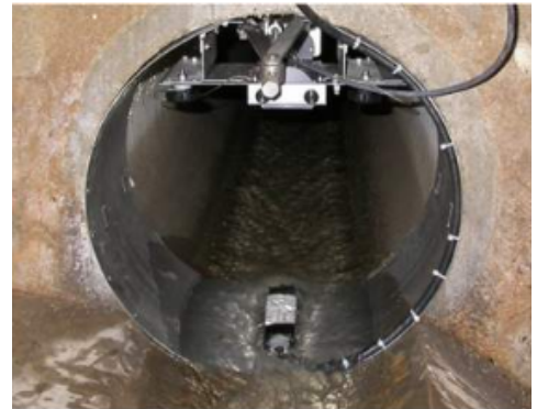
Figure 8: Area-velocity flow meter (above) and meter sensor installed in the sewer (below)
